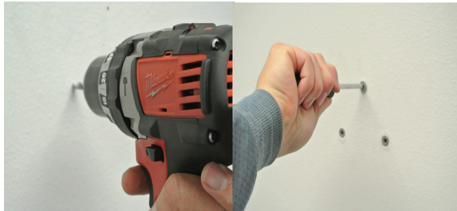
Figure 7-3 Drill and Prepare Mounting Holes
