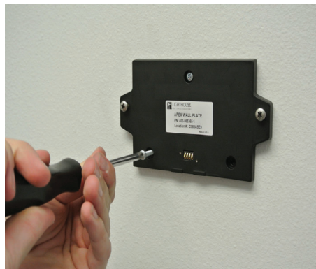
Figure 7-4 Attach SmartBracket to Wall
