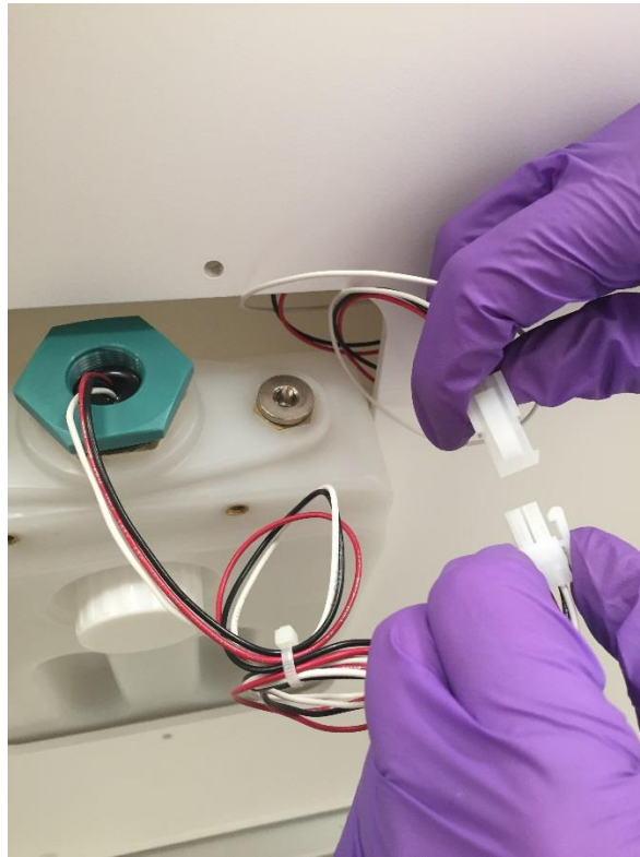
Figure 29: Water Tank electrical connector
