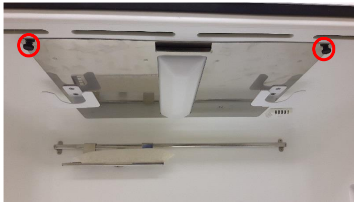
Figure 35: Ceiling Panel Thumb Screws
