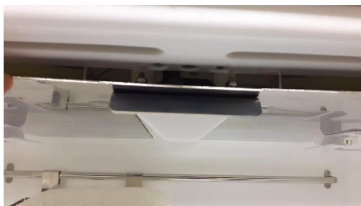
Figure 36: Ceiling Panel Handle and Grab Catch
