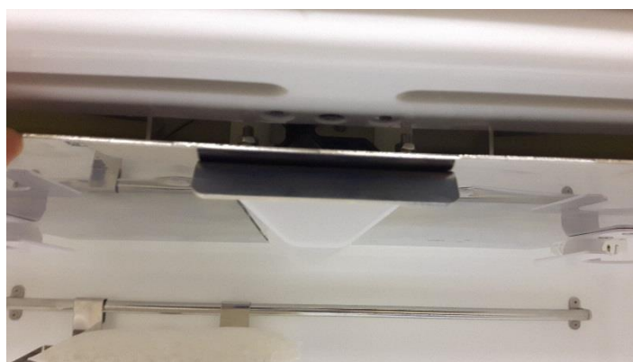
Figure 28: Ceiling Panel Handle and Grab Catch
