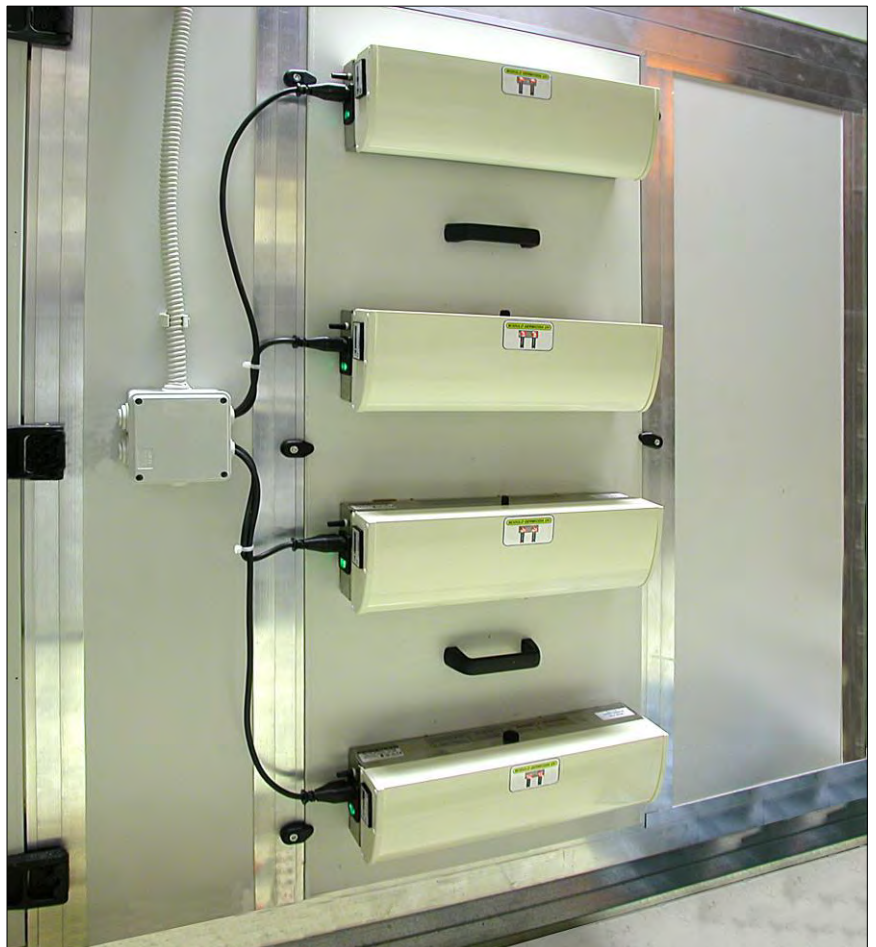
APPLICATION OF UV-DUCT-FL TO AIR HANDLING UNIT (AHU)
